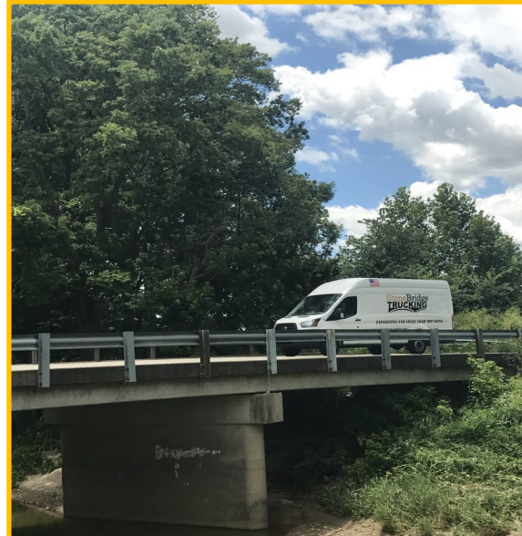
Stonebridge Transit crossing the renovated “Old Stone Bridge” outside of Greensburg, IN.
